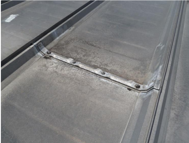
Metal Roof Deck Seam between metal panels
