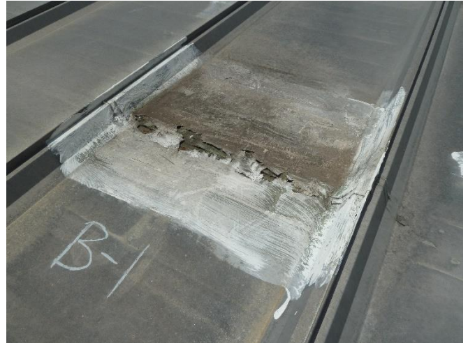
Metal Roof Deck Seam between metal panels
