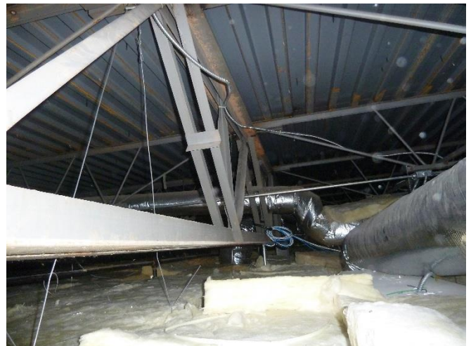
Building Structure Roof framing in office area
