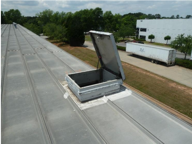
Building Structure Roof access hatch
