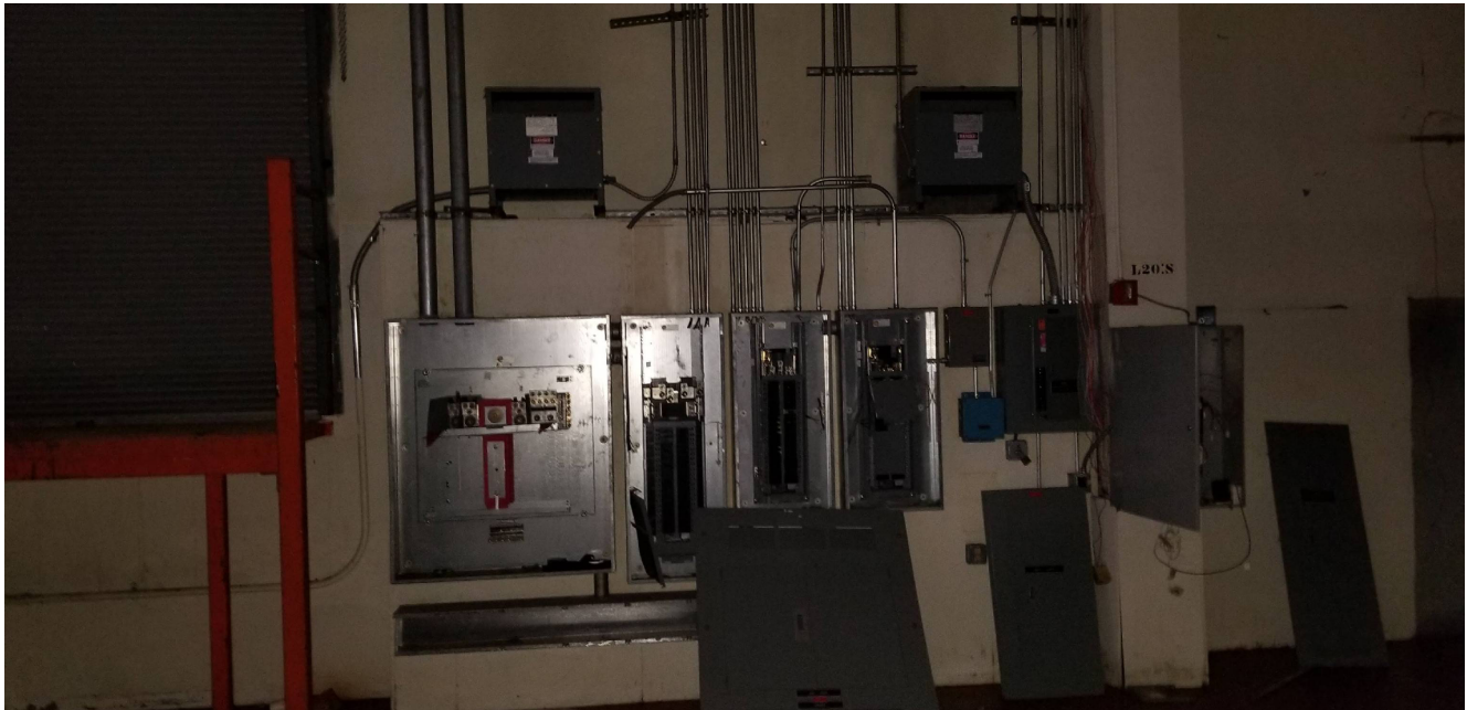
Photograph E1: Existing electrical equipment – wire stripped from panels
