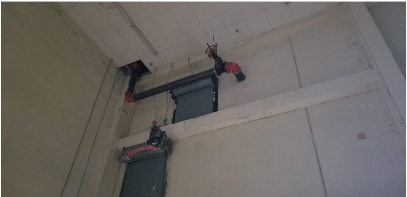
Photograph P1: Existing fire sprinkler service point from existing demolished building on West wall
