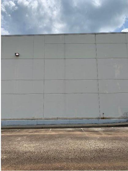
Tilt-Up Wall - Typical Warehouse surrounding walls
