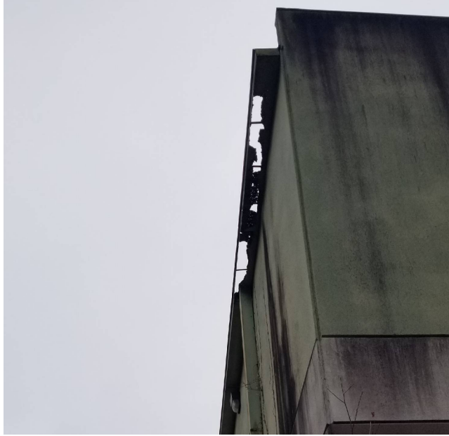
Photograph P2: Existing east wall gutter system – rusted through
