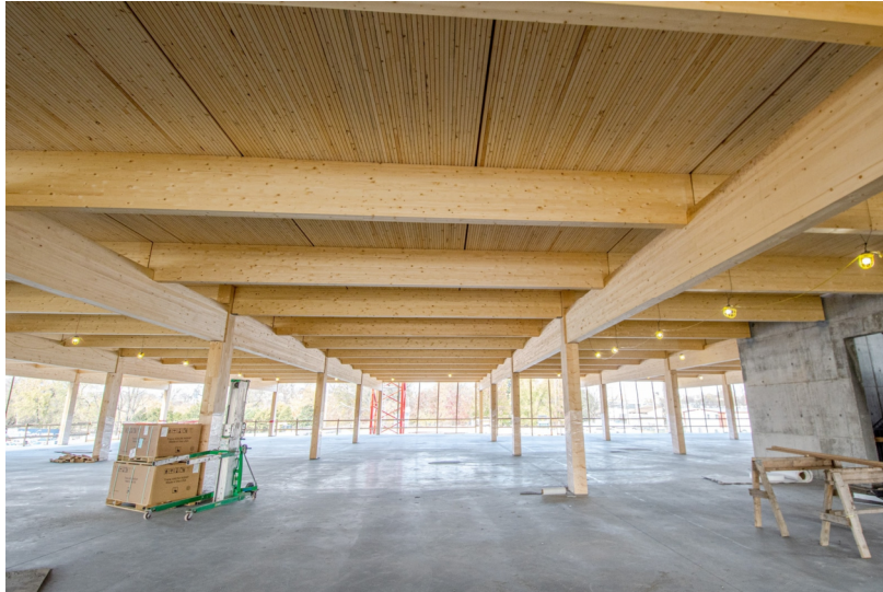
Glulam purlins and girders topped by DLT panels
