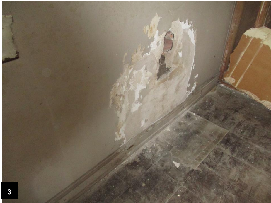
Sample 15 – Gray Wall Paint – North Wall 2 nd Floor – 1088 Murphy Avenue 0.907 wt% Pb
