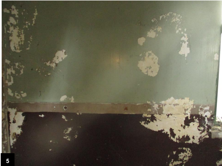
Sample 18 – Green Wall Paint – West Wall 2 nd Floor – 1088 Murphy Avenue 0.89 wt% Pb
