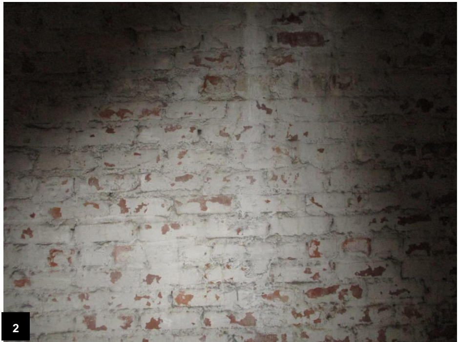
Sample 8 – White Paint on Brick – North Wall 3 rd Floor – 1100 Murphy Avenue 1.10 wt% Pb
