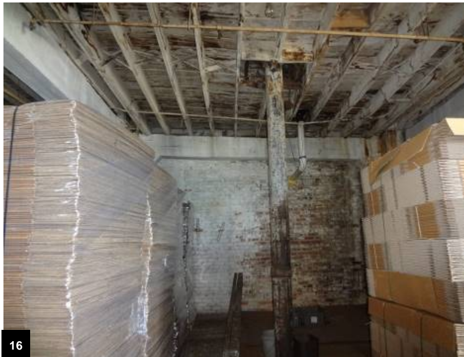
Roof penetration for water tower (empty) at Building 1088
