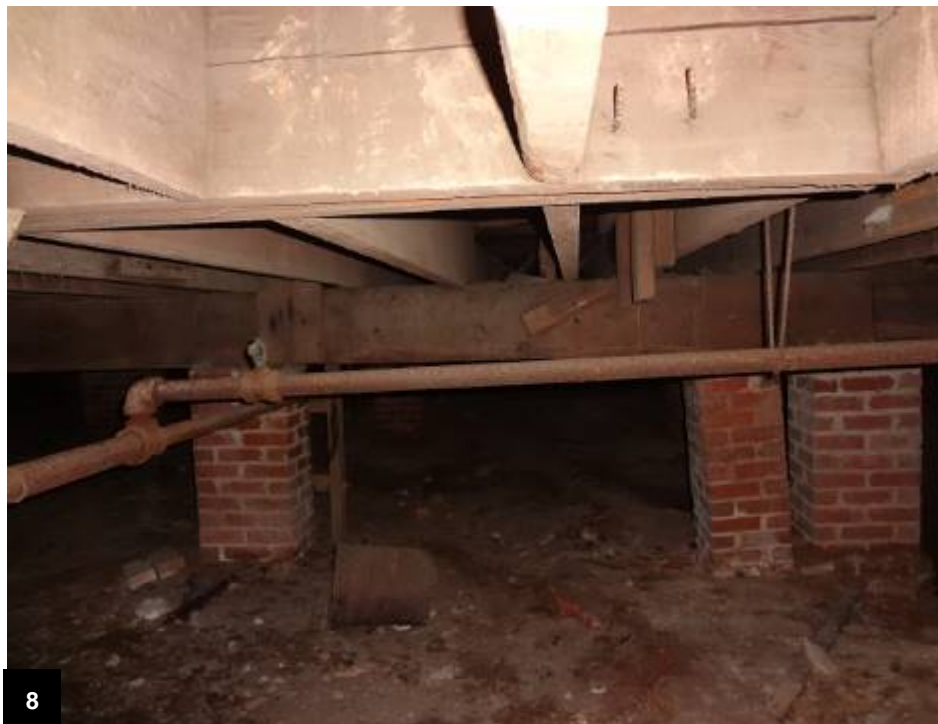
View of crawl space beneath 1088 Building
