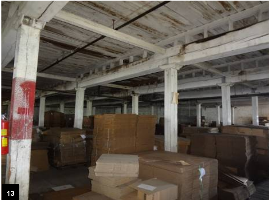
Cardboard box storage, Building 1100
