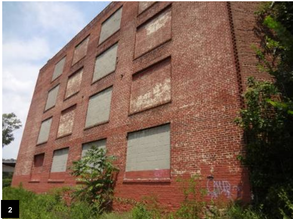
Rear elevation of 1100 Building
