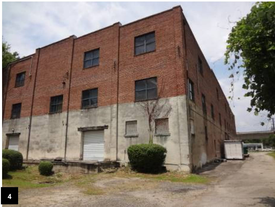
Rear elevation of 1088 Building
