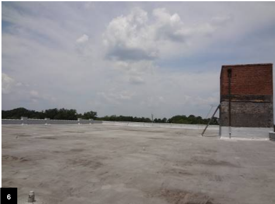
View of roof at 1100 Building
