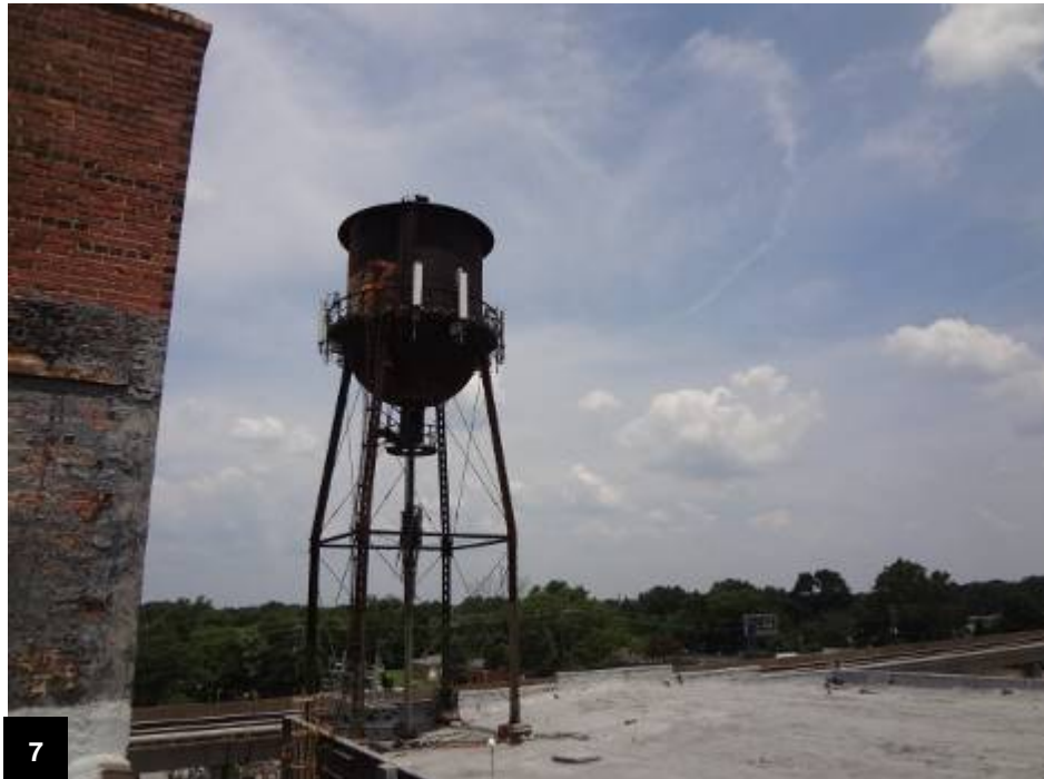
View of water tower (empty) and roof of 1088 Building
