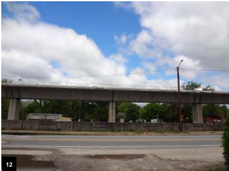
Adjacent western properties
