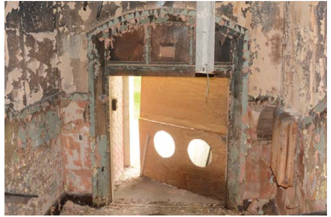
Figure 24. Arched wood windows above west entry door.
