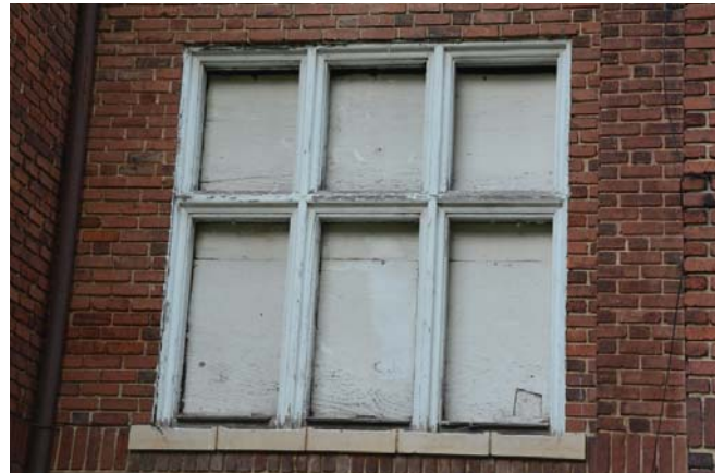
Figure 25. Wood window frame at first floor of 1911 building.
