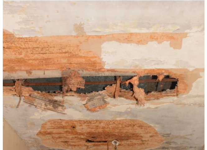
Figure 63. Plaster ceiling on expanded metal lath.
