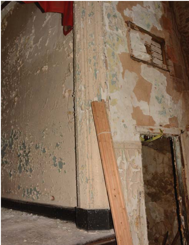
Figure 19. Detail of proscenium arch.
