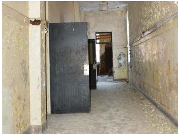
Figure 78. Non-historic interior flush door.
