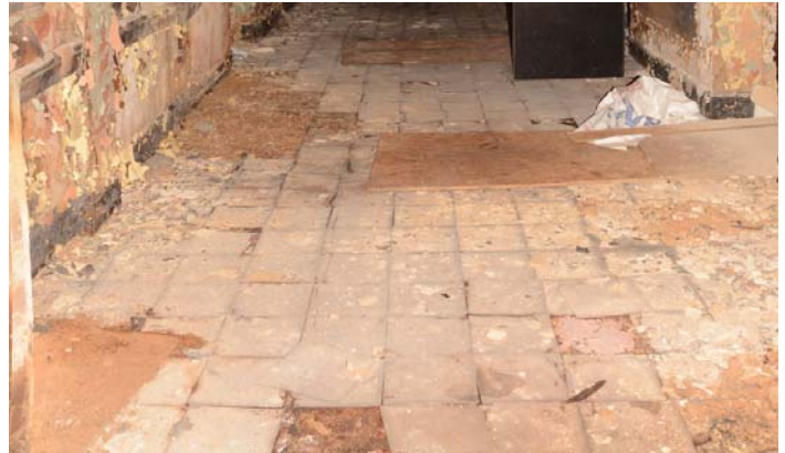
Figure 59. 9x9 VAT flooring over wood floors in the corridor.
