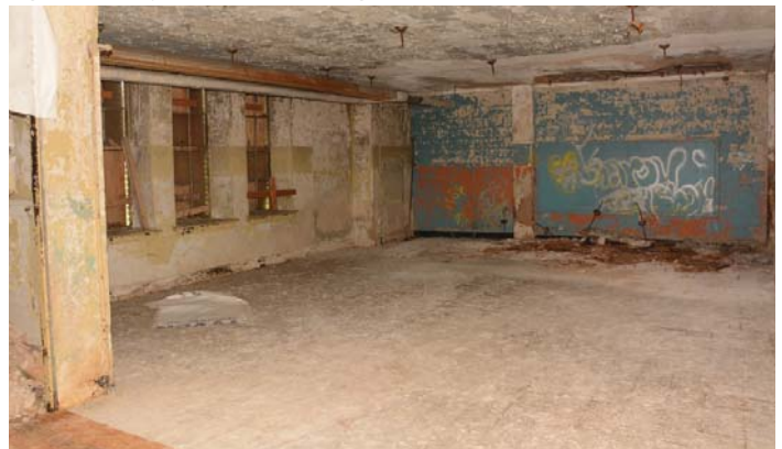
Figure 61. Concrete floors in the wings are generally in stable condition.
