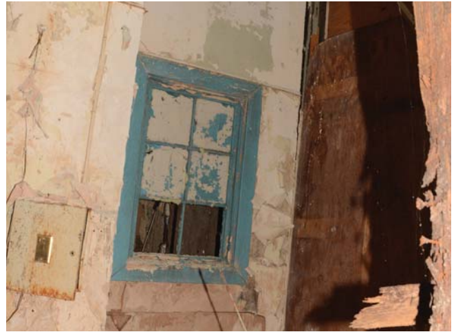
Figure 28. One-off six-lite interior window.
