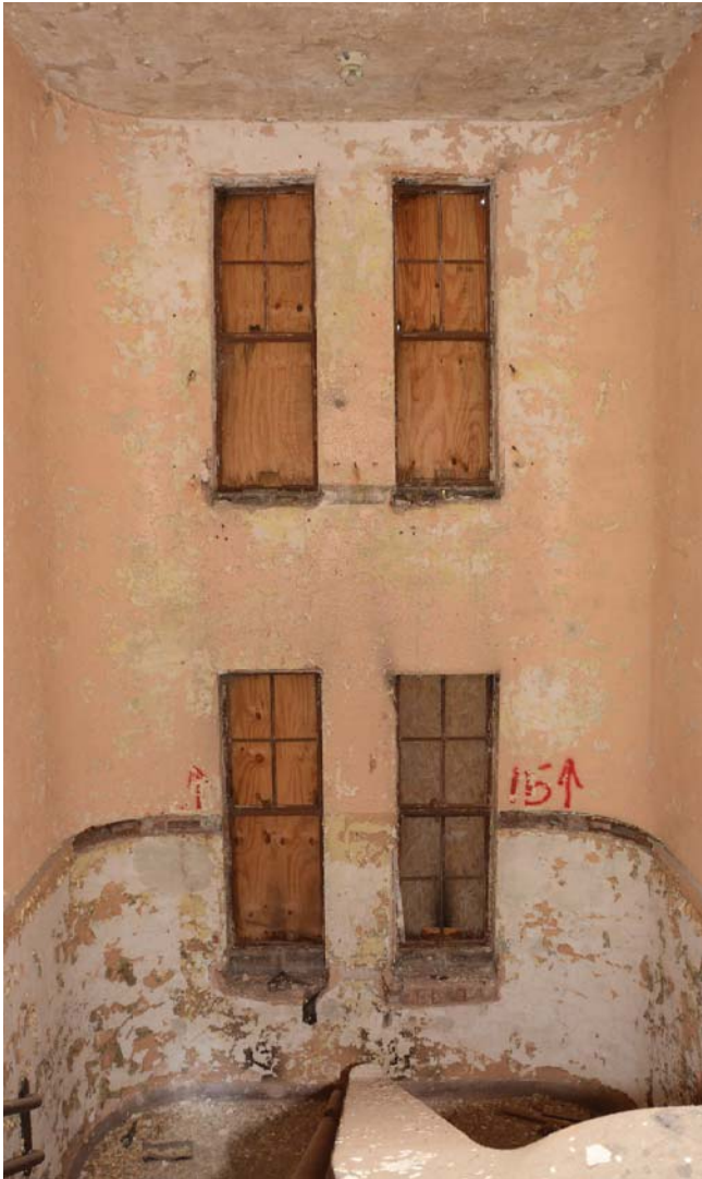
Figure 71. Steel windows at stair towers.
