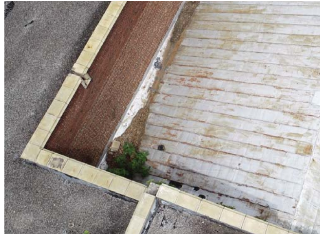
Figure 54. Auditorium roof at intersection with the south wing.
