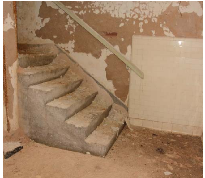
Figure 81. Concrete stairs leading to Auditorium.
