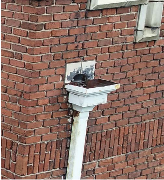
Figure 16. Scupper, collector head, and downspout on the 1911 portion of the building.
