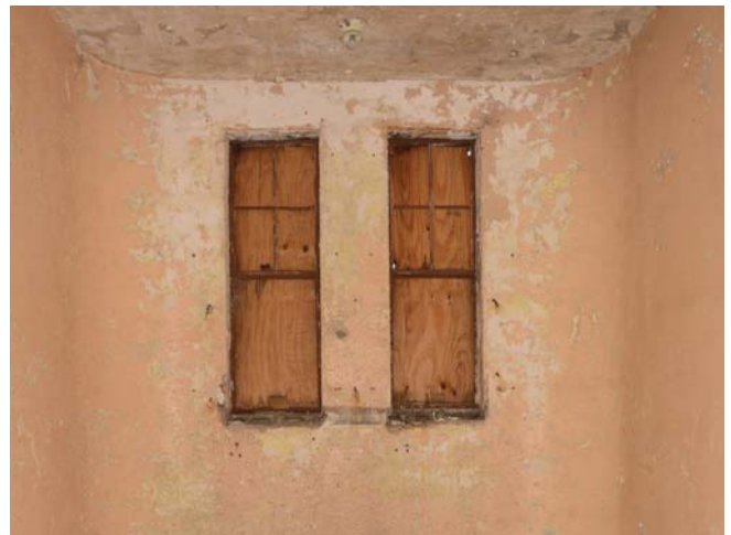
Figure 30. Typical stair tower steel windows.
