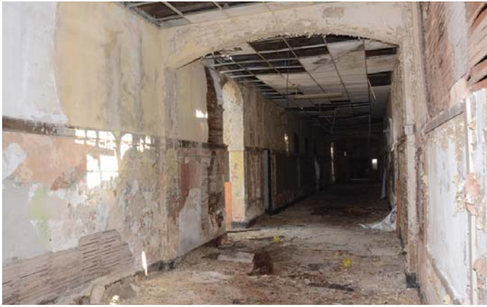
Figure 56. Typical condition of corridor walls.
