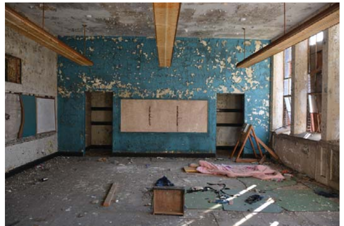
Figure 20. Typical flat plaster walls in 1923 wing classroom.
