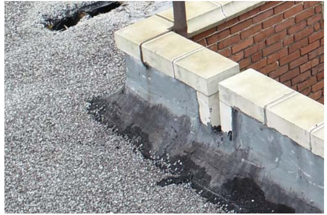
Figure 53. Terracotta parapet with built-up flashing
