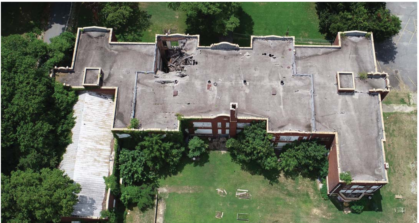
Figure 55. Overall view of the roofs.
