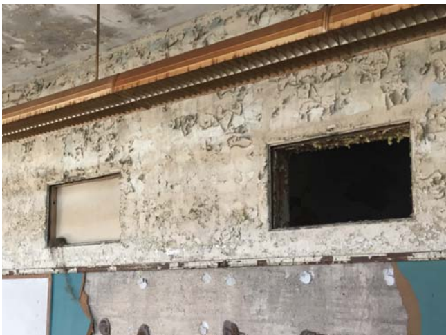
Figure 72. Interior transom windows
