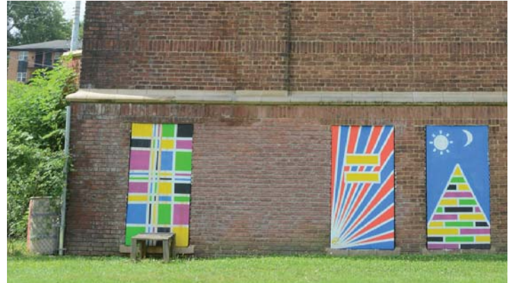
Figure 10. Infill brick on north elevation.
