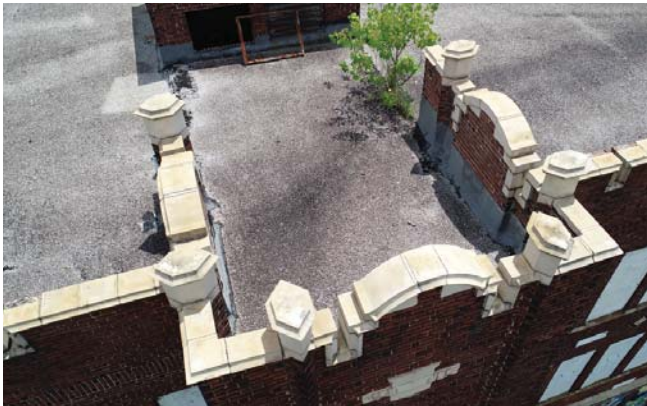
Figure 13. Detail of decorative terra cotta coping.
