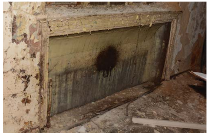
Figure 40. Radiator recess in Auditorium.
