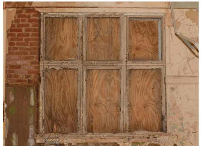
Figure 74. Wood window frame.
