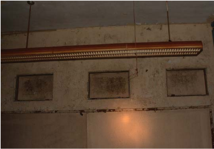
Figure 27. Boarded up windows facing corridor.
