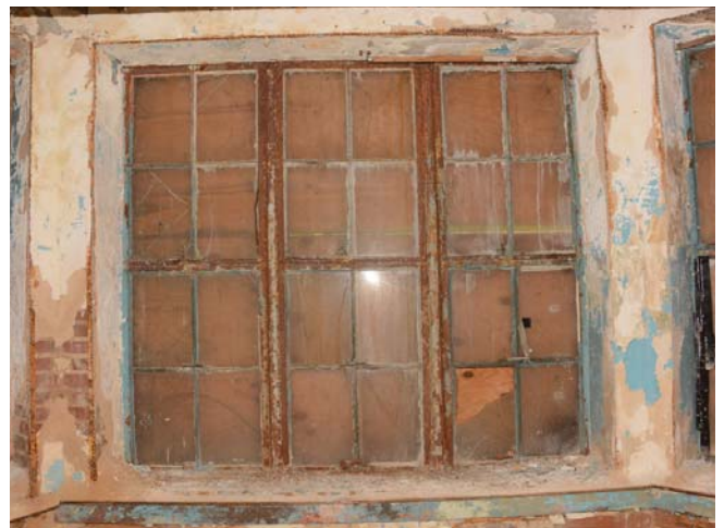
Figure 75. Steel windows in the bay window at the basement level.
