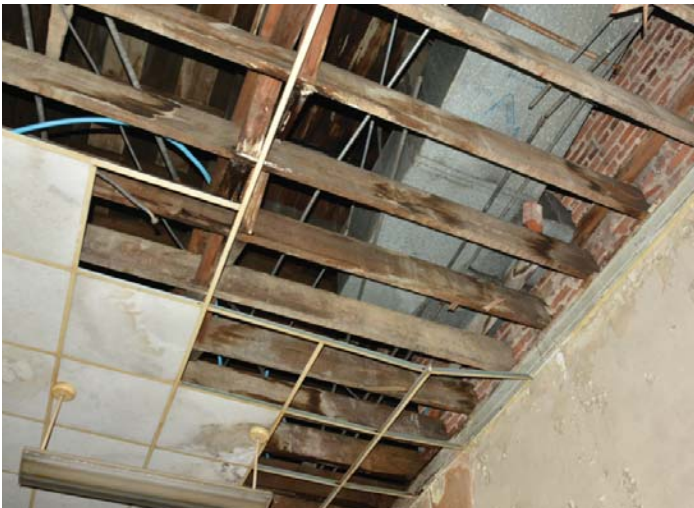
Figure 82. Old Mechanical Ducts in Ceiling at Third Floor
