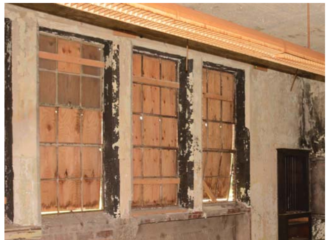
Figure 32. Portion of a typical bay of classroom steel windows.
