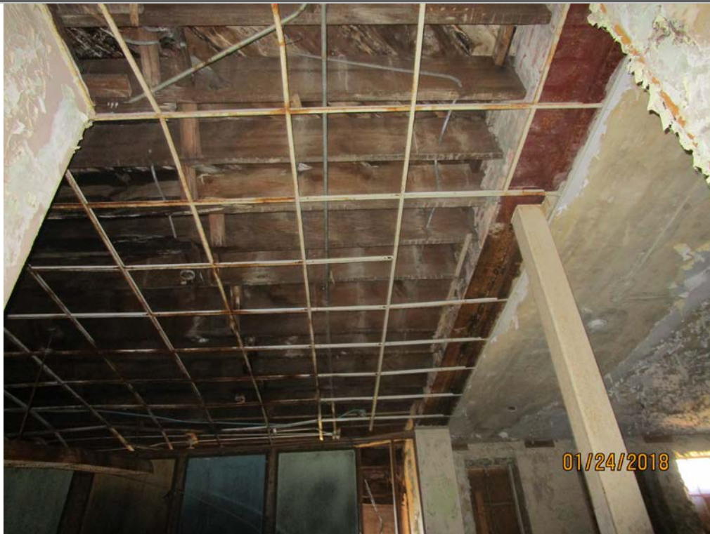
Steel support beam.
