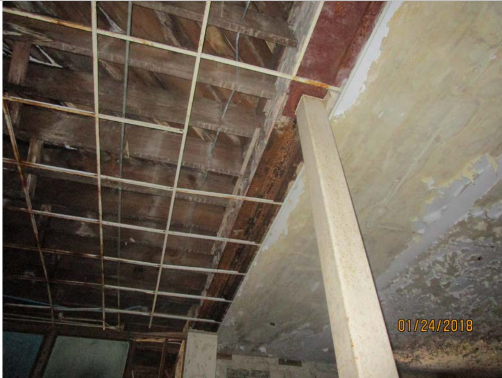
Steel support beam.
