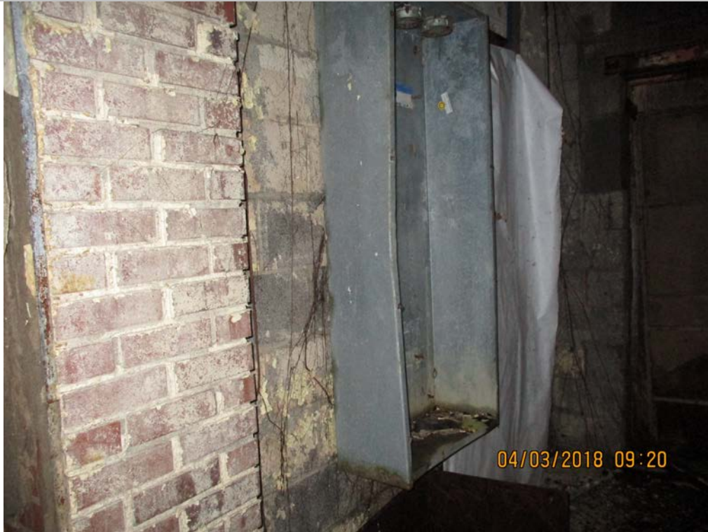
CMU block foundation wall in good condition.
