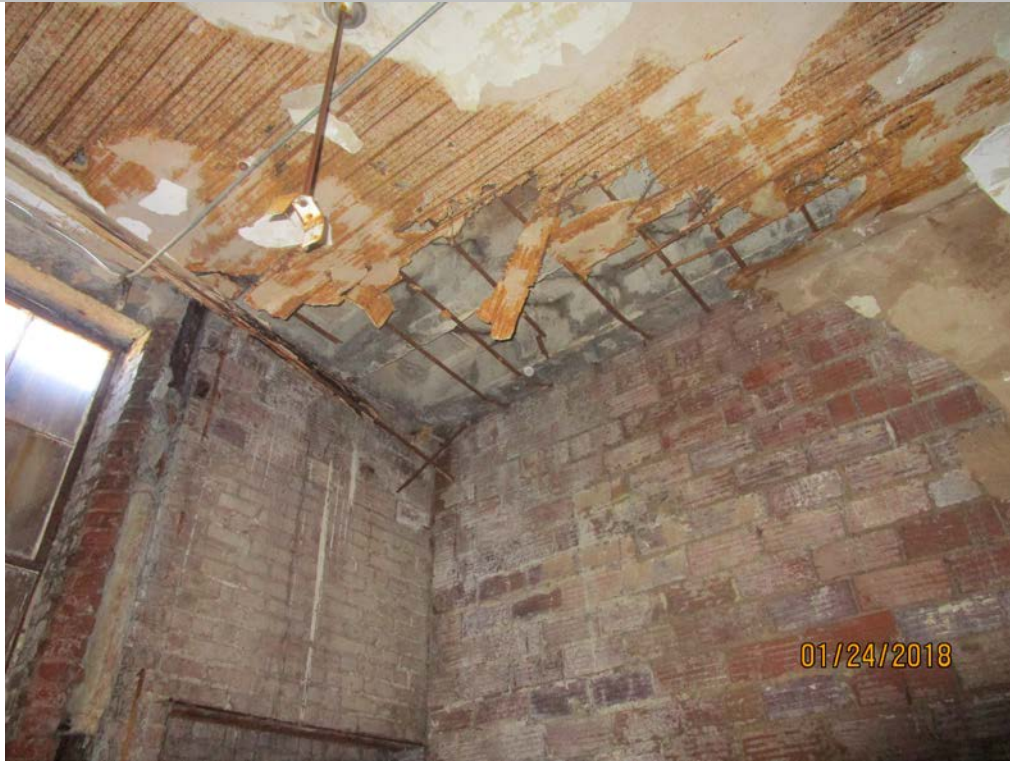
Concrete floors with plaster underneath.
