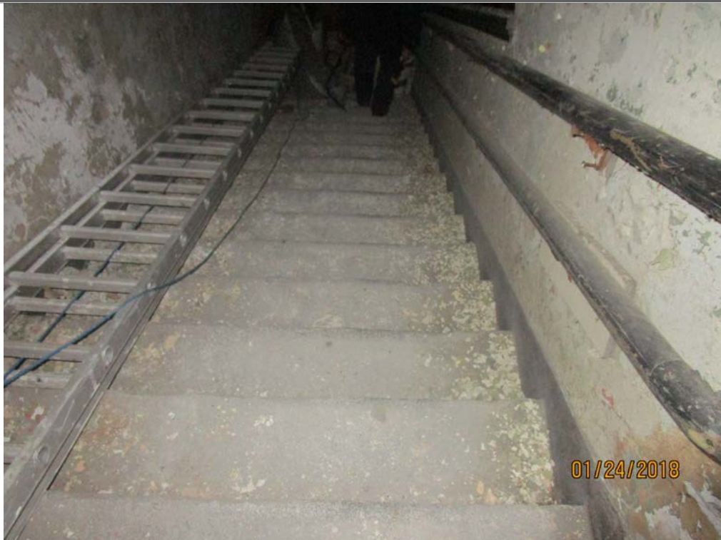
Concrete stairs are in good condition.
