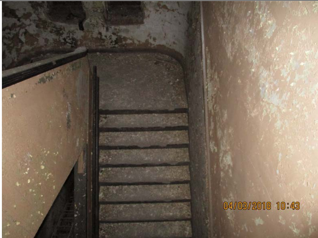
Concrete stairs are in good condition.
