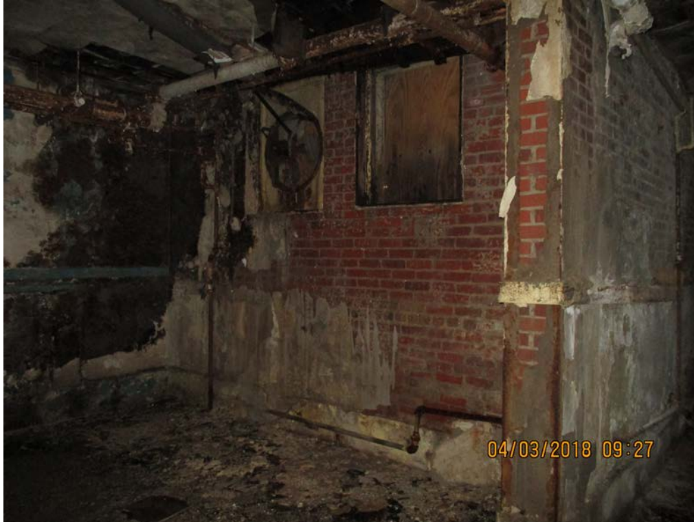
Structural brick foundation wall that is in good condition.
