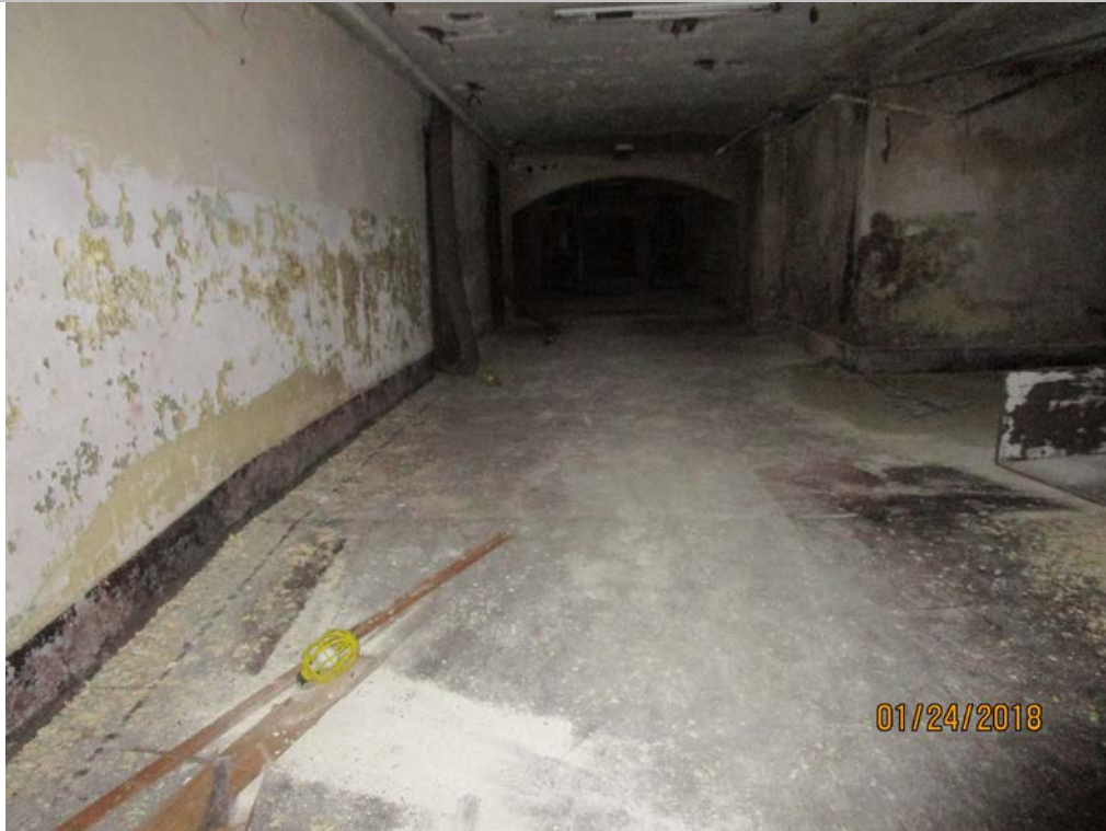
Concrete slab at basement level is in good condition.
