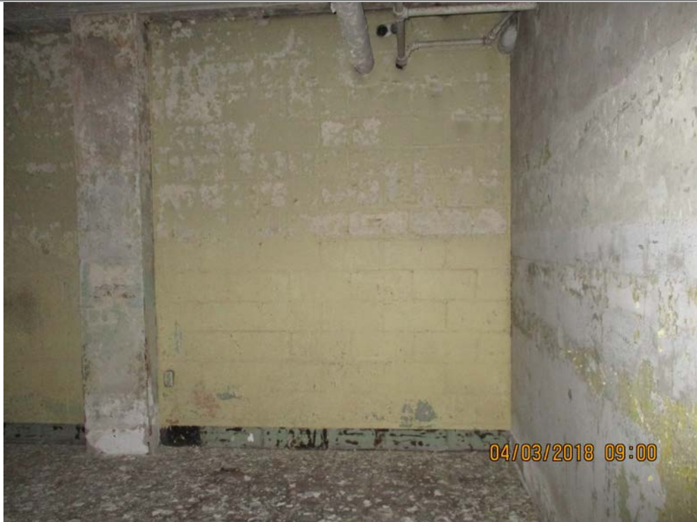
Interior CMU block wall.
