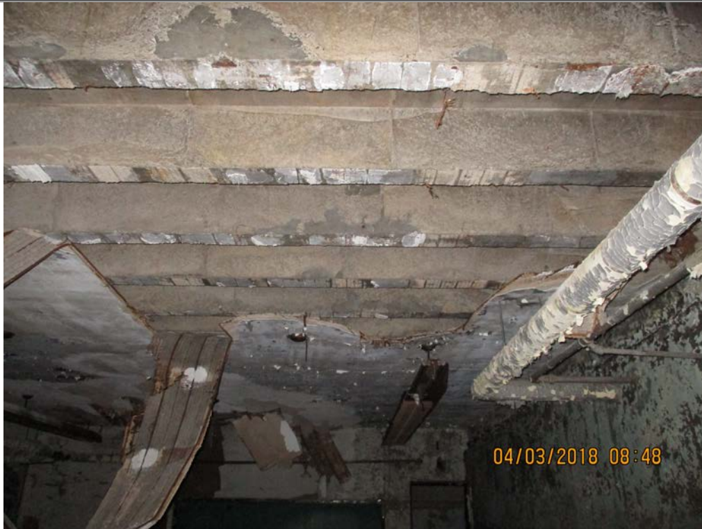
Concrete floors covered with plaster underneath.
