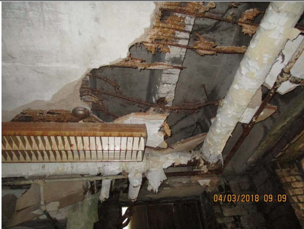
Concrete floors with plaster underneath.
