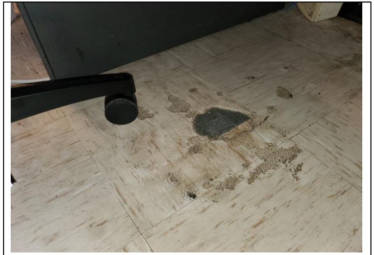
4. 9" x 9" Floor Tile/Mastic under 12" x 12" Floor Tile
