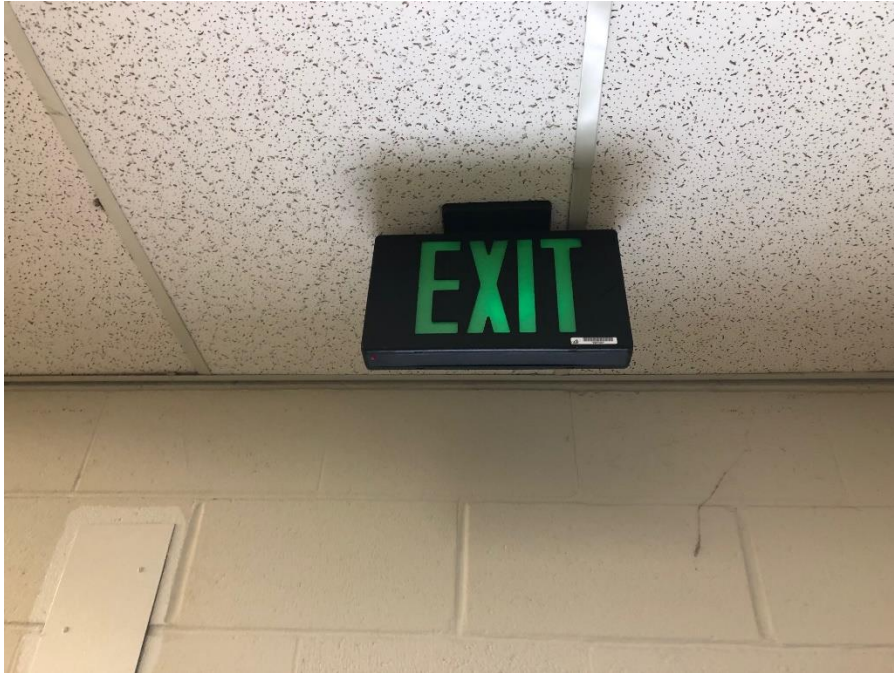
Photograph 3: Typical view of the emergency exit signs located at the Subject Property.
