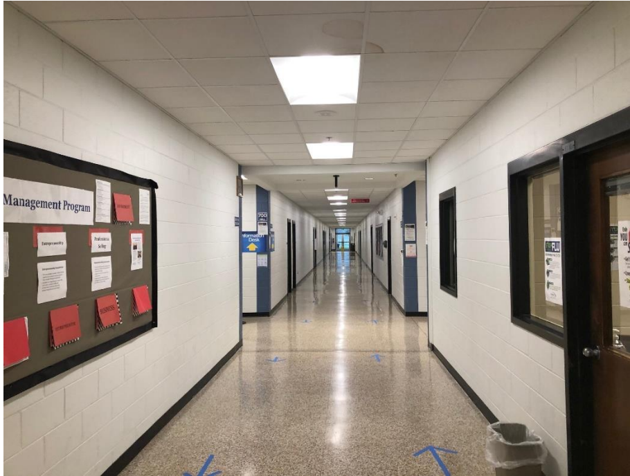
Photograph 1: Typical view of the Fluorescent light ballasts located at the Subject Property.
