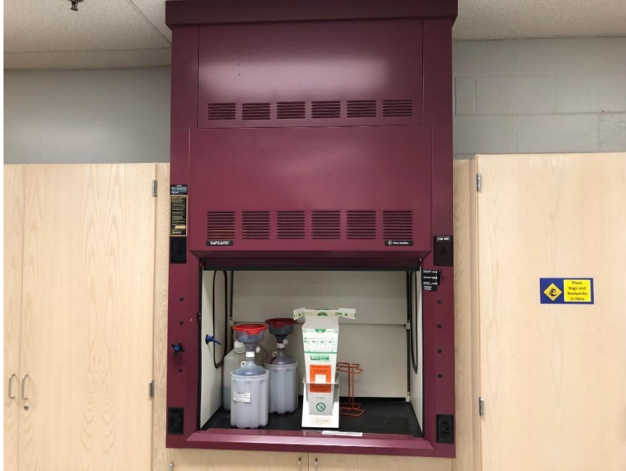
Photograph 9: Typical view of the chemical vent hood located at the Subject Property.
