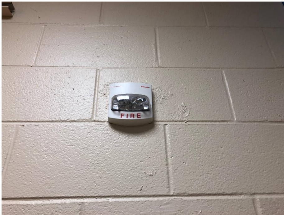
Photograph 4: Typical view of the High Intensity Discharge (HID) lighting located at the Subject Property.
