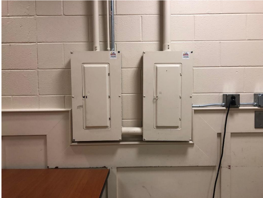
Photograph 7: Typical view of the panels/breakers located at the Subject Property.
