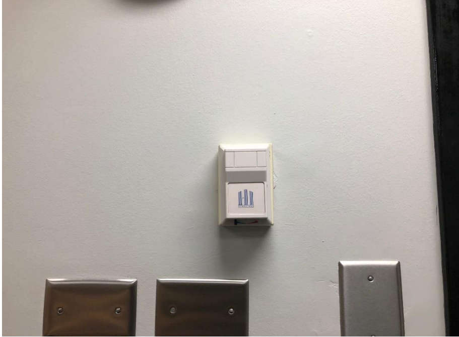
Photograph 5: Typical view of the thermostats located at the Subject Property.
