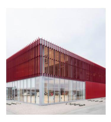
Metal Louver System Project goal adjustable metal louvers. BOD Alucobond - Alufoil Provide coordinating metal wall panel for small section of wall on North Elevation
