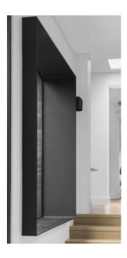
Interior punched openings. Labeled as "Window A" on plans to be low profile black frame cased with offset steel plate casing. Similar look above.
